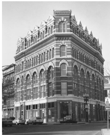
Vacant for many years, the Rice Building in downtown Troy, was redeveloped by a partnership of the Troy Savings Bank, Rensselaer Polytechnic Institute, and the Troy Architectural Program, Inc. The building is now fully occupied and used as a high-tech "incubator."
