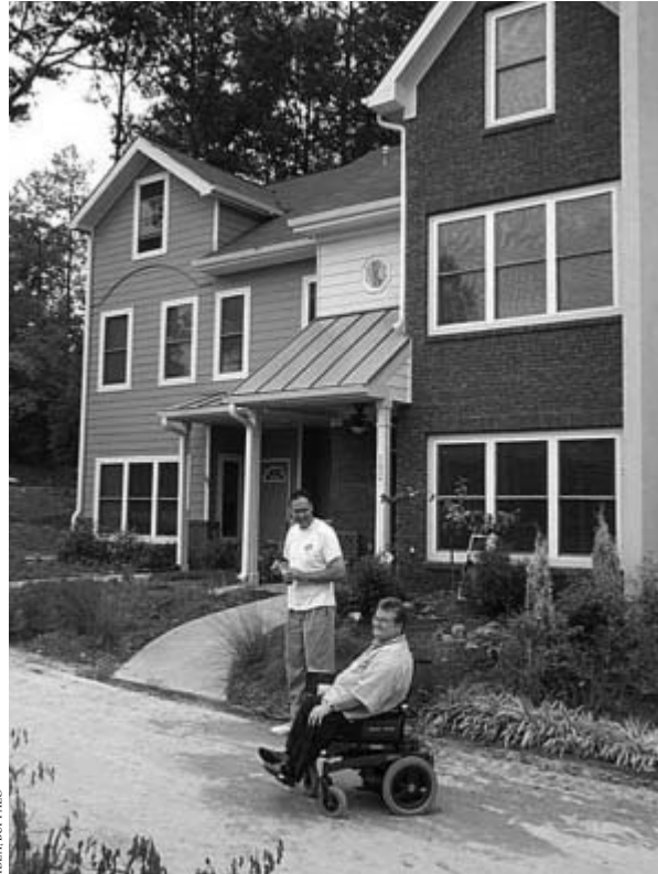
No step entries help make housing accessible to a diverse population, including people who use wheelchairs.
